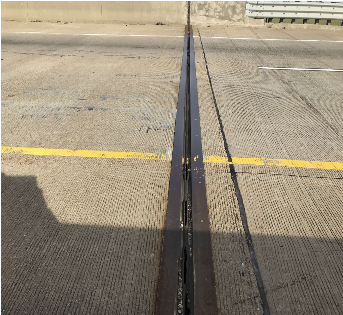
PHOTO 1 Description Abutment #2 joint material has 50% torn.
