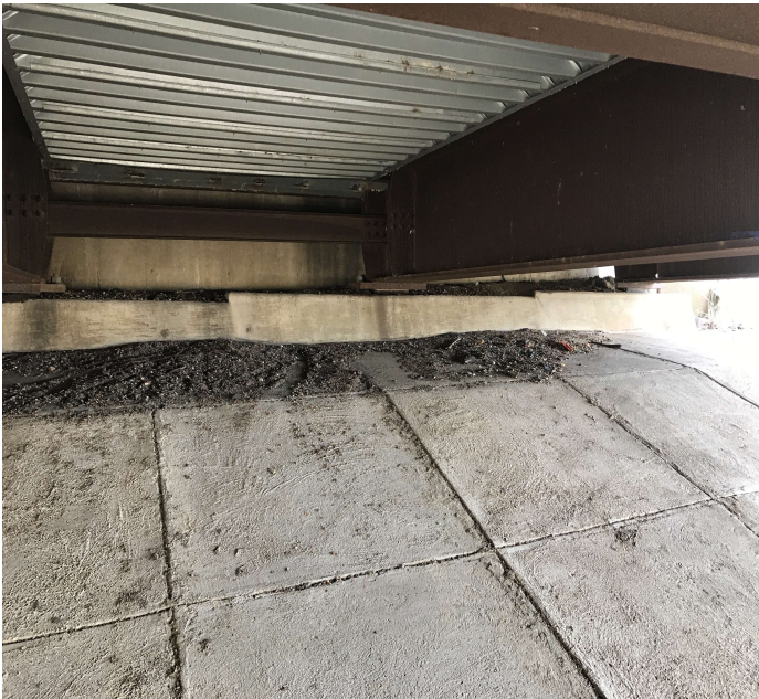
PHOTO 1 Description Abutment #1 cap has dirt and debris on it.
