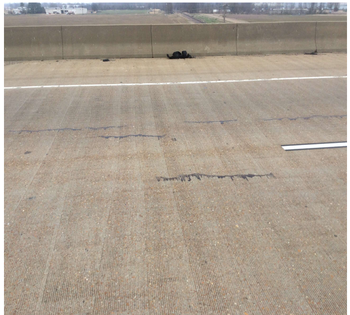
PHOTO 2 Description Typical sealed longitudinal deck cracks (3 sealed 3 unsealed) full length
