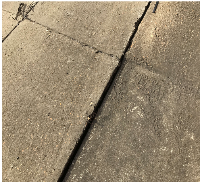
PHOTO 2 Description Abutment #1 slope right side has a voided area under slope pavement.
