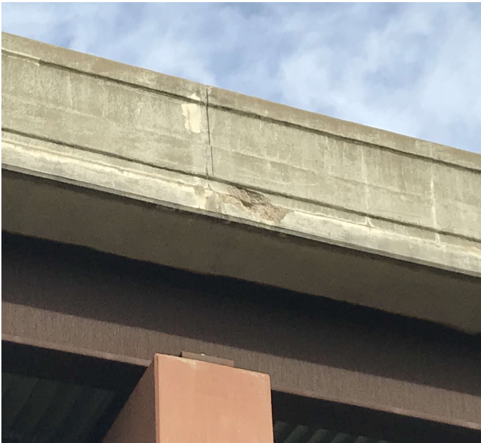
PHOTO 1 Description Spall at bent #3 right side outside of wall.
