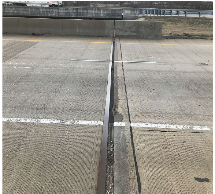
PHOTO 2 Description Abutment #1 joint material has six small torn areas.
