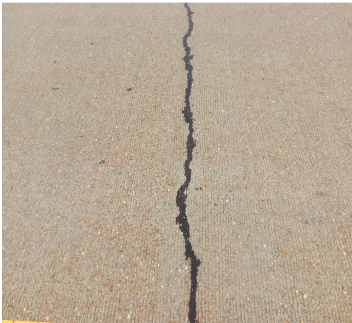
PHOTO 1 Description Typical sealed transverse deck cracks
